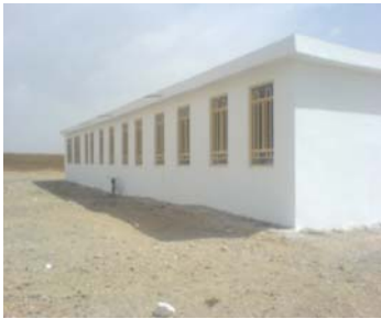
Newly constructed School building in Helmand Province
