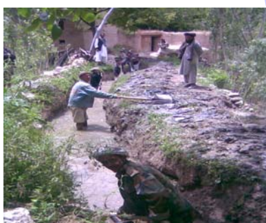
Ditch Cleaning in Samangan province under CBDRR
